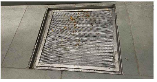
FIXED SS PERFORATED SHEET
