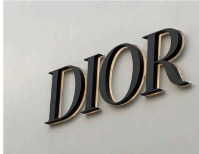
SS / Metal cut letters backlit in shade matching ss used in double height portal.
