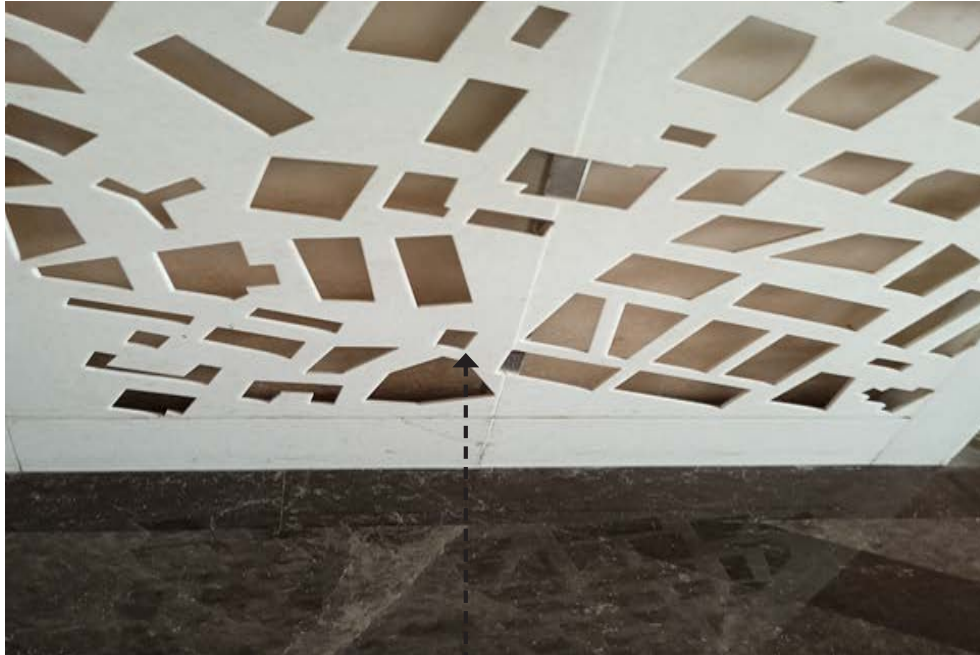
Corian Marble in MALS is chipped at many places, need repair work.
